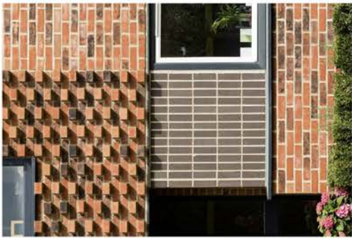
PRECEDENT: FLEMISH BOND DETAILING, HORSTEAD PARK, KENT BY PROCTOR & MATTHEWS ARCHITECTS
